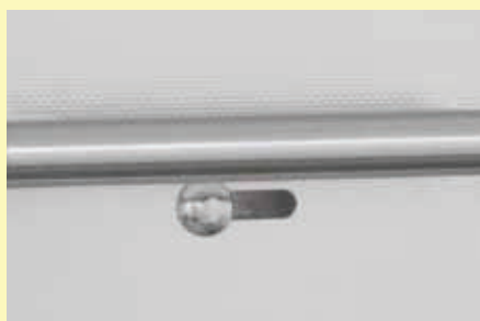
Adjustable air inlet integrated in the door
